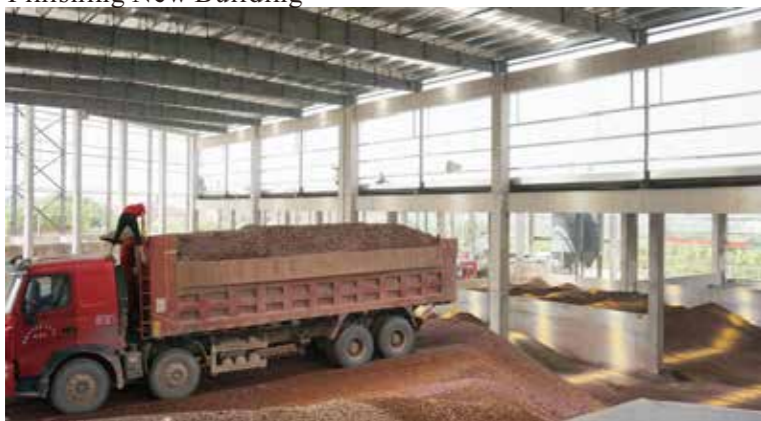
全封闭商混材料仓 Closed Commercial Concrete Store Area
