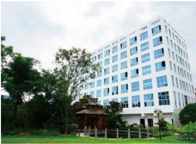
即将竣工的新大楼 Finishing New Building
