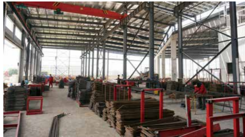
新的钢筋加工棚 Reinforcement Processing Plant
